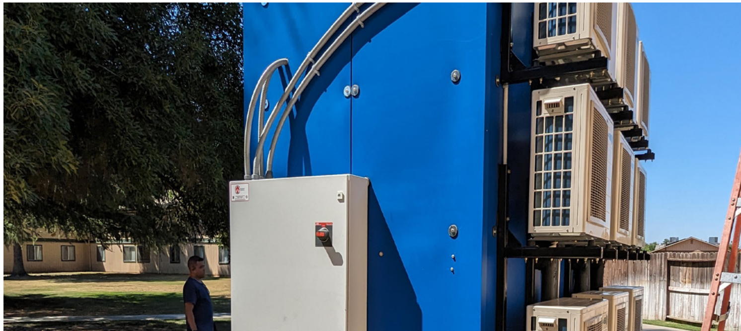
Outdoor WaterDrop packaged central heat pump water-heating system. Image source: Carbon Zero Buildings / BetterBricks.
